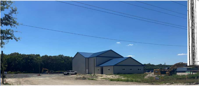
Lot #11- 250 Garrison Oak Drive BHD Operations Facility – Under Construction
