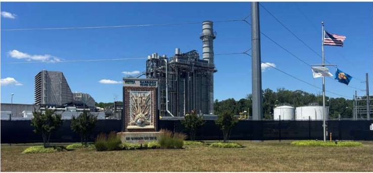
Lot #7- 450 Garrison Oak Drive Garrison Power Plant
