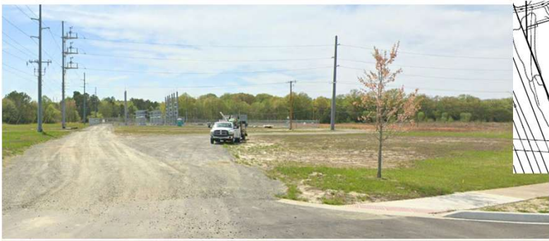
Lot #14- 100 Garrison Oak Drive City of Dover Substation – Built to Accommodate Park Needs
